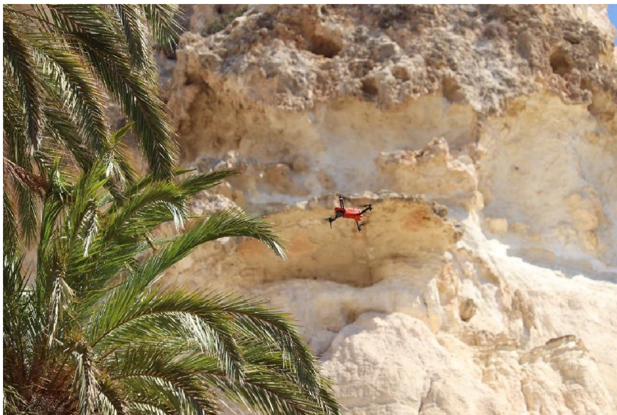
Figure 14: Visual inspection with aerial unmanned vehicles
